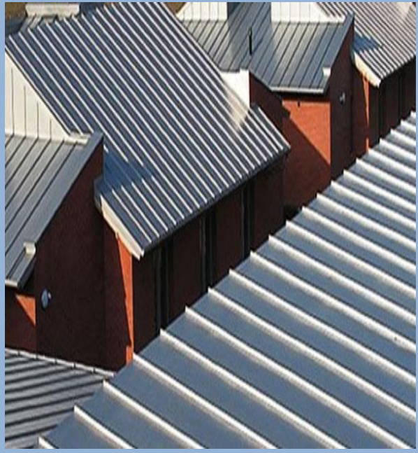
STANDING SEAM ROOF
