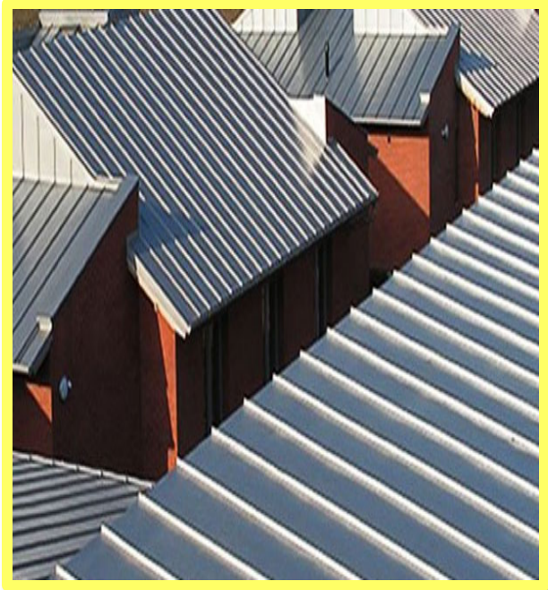
STANDING SEAM ROOF
