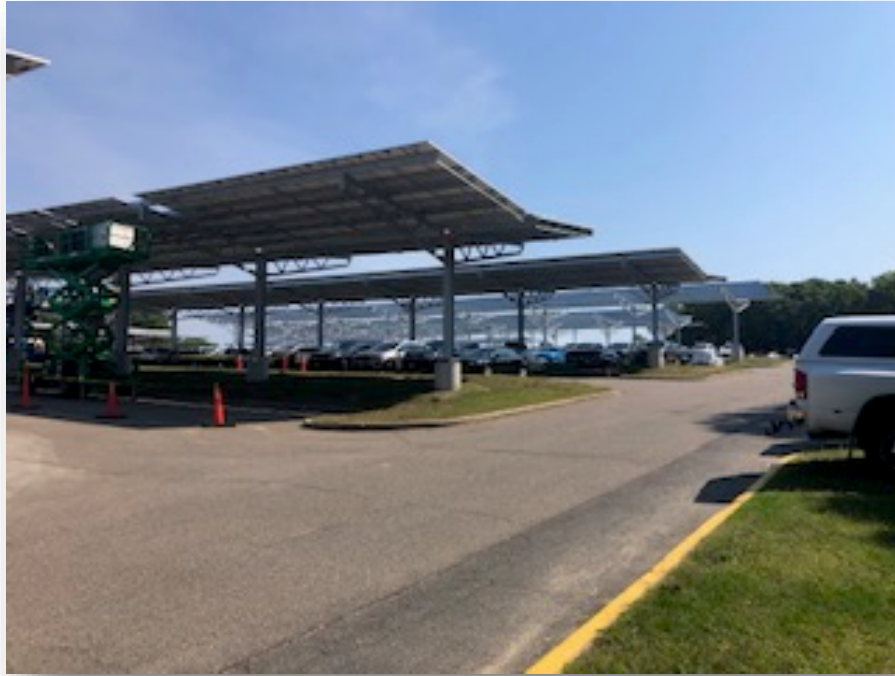
Renewable Energy – Photovoltaic Electric Generation (Solar Canopy / Carport System)
