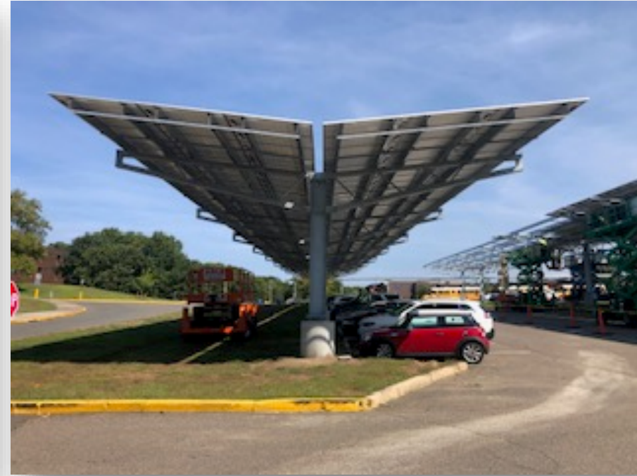
Renewable Energy – Photovoltaic Electric Generation (Solar Canopy / Carport System)
